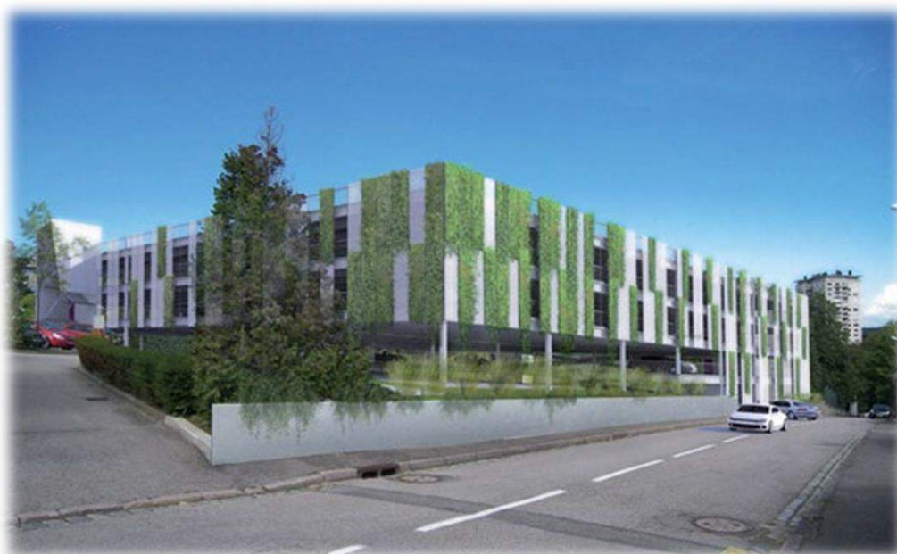
Parking silo, Epinal
